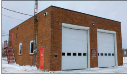
The Billings firehall will be demolished with a new one built in its place.
