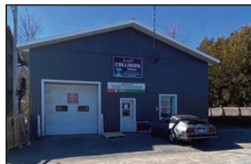
Mechanical Garage Building & Business MLS®#: 2092721, $499,000
