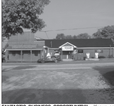
FANTASTIC BUSINESS OPPORTUNITY!! - Known as Sandfield General Store, this very large commercial building is currently a gift shop, a restaurant & a corner store. It has plenty of parking, storage areas & land. Along with this business is a 2 storey, 5 bdrm, 2 bath home that would make a great little bed & breakfast. Lake Manitou is a stone's throw away & this location is quite central & very much needed as the competition is mainly 20 mins or more away in every direction. There is a resort trailer park directly behind this great commercial business & its huge untapped potential. Asking $395,000. MLS#2062706
