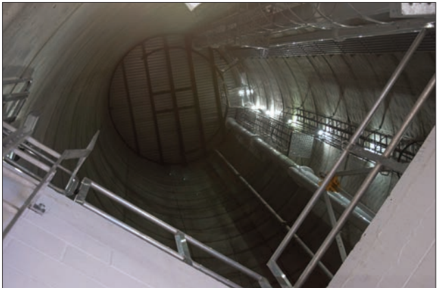
Look way up! From the base of the elevated storage reservoir, a cavernous tower separates the water tank from the ground. Water enters the structure with 100 pounds of pressure and its high elevation ensures consistent water pressure for the entire area.
