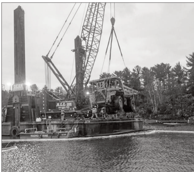
A crane removes a dump truck from the Killarney Channel.
