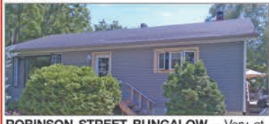
ROBINSON STREET BUNGALOW - Very attractive Little Current home in a highly attractive location with spectacular landscaping, mature hardwoods & huge rear yard with great privacy. Major renovations include siding, most windows, re-tiled basement & new propane furnace. Features include 3 bdrms, large rear deck & full unfinished basement. Great price at only $189,900. MLS#1028178
