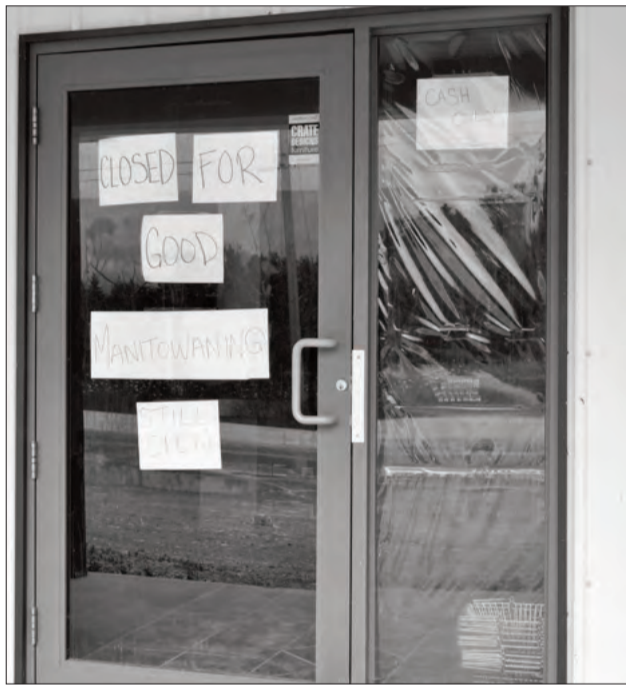
The sign on the door at Barney's Bargain Barn Home Store reads 'closed for good' following the eviction notice by the Northeast Town. Barney's is one of six tenants located at the 'unsafe' building.
