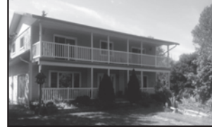
CENTRALLY LOCATED LITTLE CURRENT HOME
