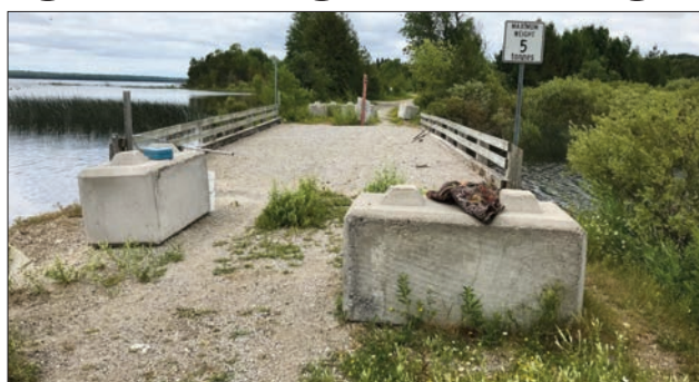
The Rogers Creek bridge has been closed since 2015.
