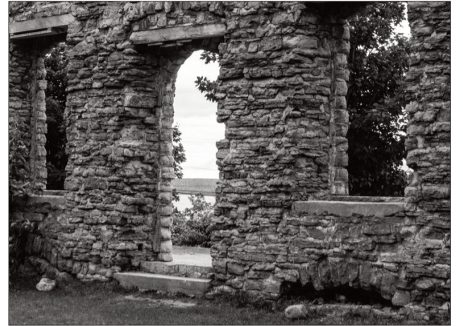
The Jesuit Mission in Wiikwemkoong built a church and residence on this site in 1849, both of which burned in 1954; the church was rebuilt while these ruins of the former school and residence are now home to the summer productions of Debajehmujig theatre group.
