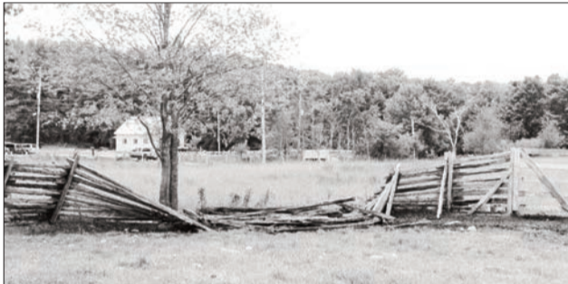
A portion of fence lays flattened from the force of the microburst's winds.
