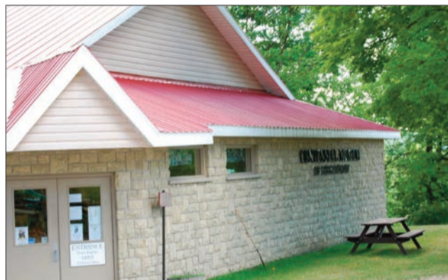
The Centennial Museum of Sheguiandah will see new displays this summer.
