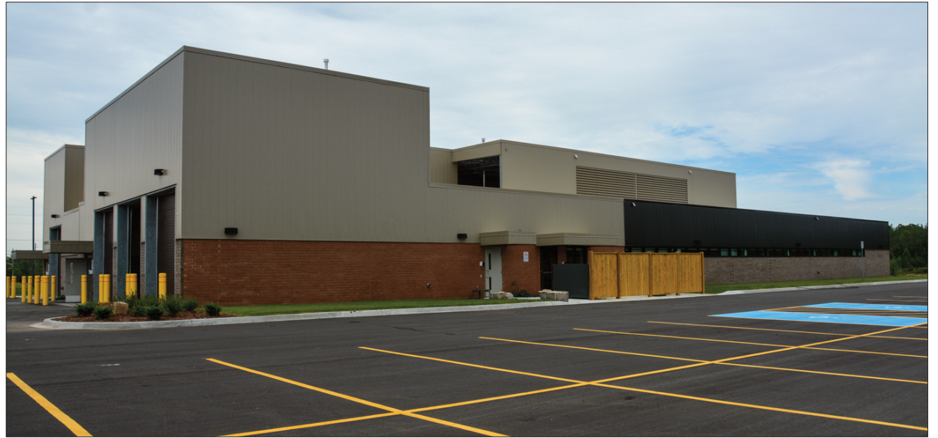
A view from the 'police only' parking lot located on the north side of the new detachment in Little Current.
