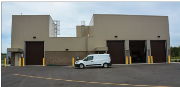
The left bay is for prisoner transport while the three bays on the right are for cruiser maintenance.
