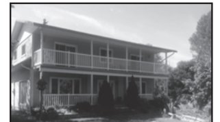
CENTRALLY LOCATED LITTLE CURRENT HOME
