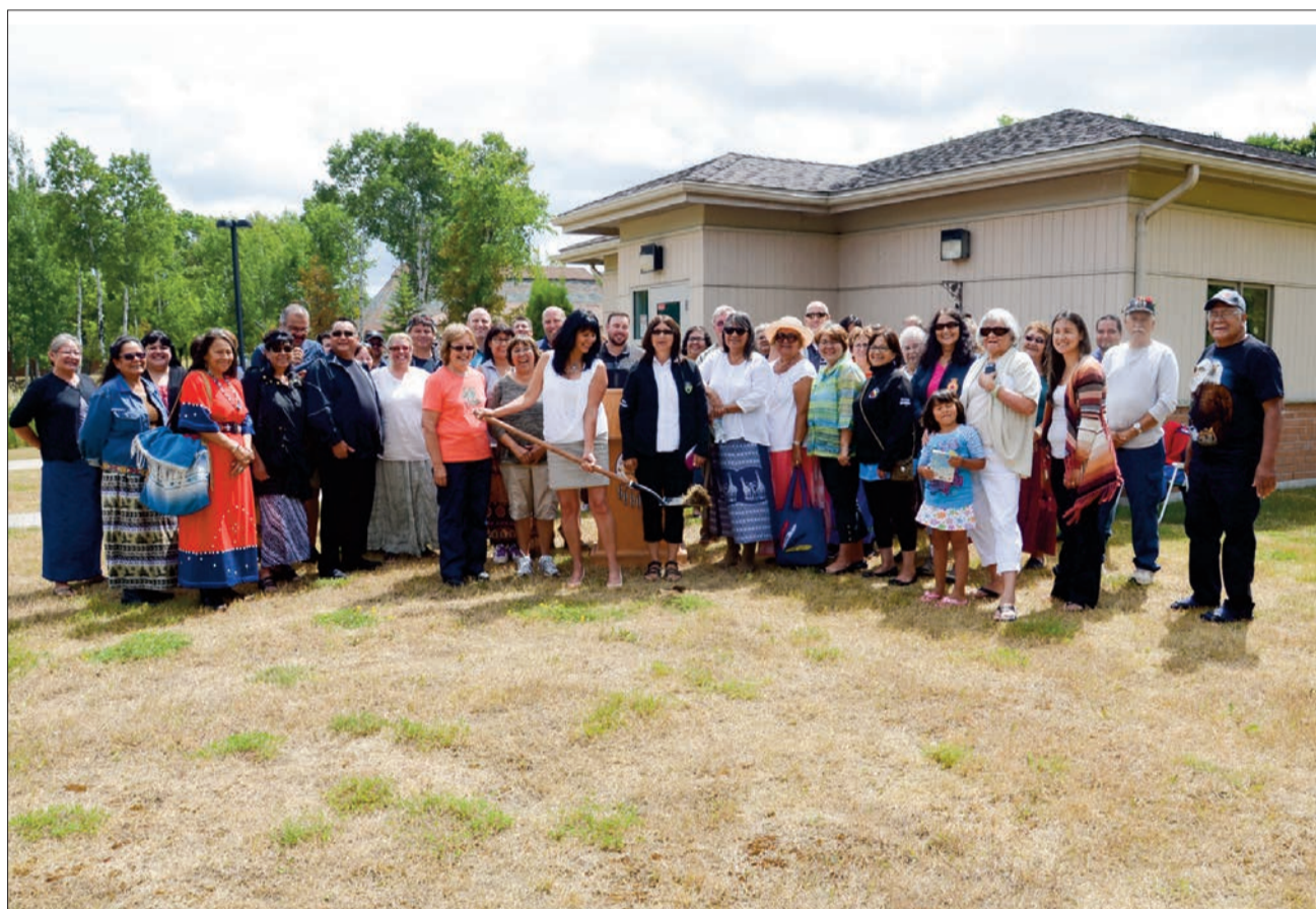
A jubilant Noojmowin Teg Health Centre Executive Director Pamela Williamson wields the shovel during a ground-breaking ceremony announcing $2.36 million in funding from the Ontario Ministry of Health and Long-term Care for a new expansion of the building which houses both Noojmowin Teg and Mnaamodzawin Health Services Incorporated. The new building will include expanded facilities for 15 health care professionals as well a healing lodge, space for medicines and making of medicines, a healer clinic space, medical examination room, two mental health counselling rooms, as well as a large space for meetings and workshop activities.
