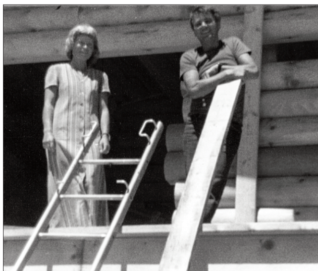
The whole family helped build the house on Dominion Bay.
