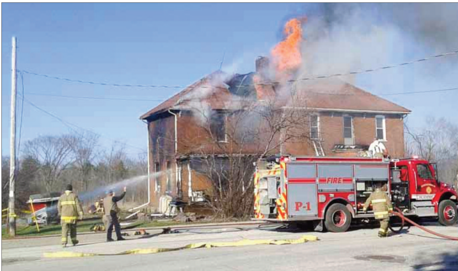
A piece of Manitowaning history was lost to fire Saturday night. Assignnack firefighters worked feverishly to save the century home, but the blaze was too much and the house, which was under renovation by its owners, was completely lost.
