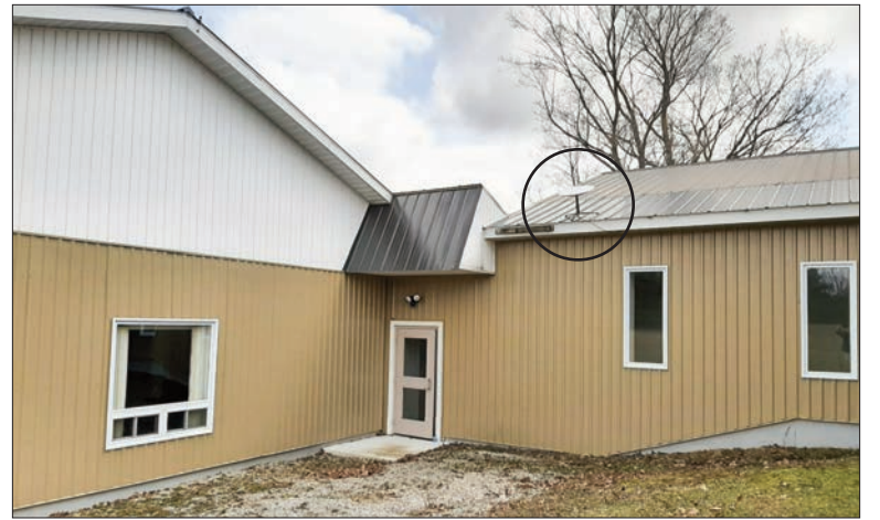
A small microwave dish atop the Tehkumma municipal office powers the building with much faster internet speeds. (Dish is circled.)
