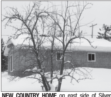
NEW COUNTRY HOME on east side of Silver Water being 1120 sq. ft. w/2 bedrooms, full bath, utility room & open area for kitchen dining living. Just built last fall, this work in progress, is finished to the vapour barrier w/200 amp service, electric & wood heat, full crawl space, drilled well & septic. Except for some furniture, everything stays including building materials, all construction tools, 5 appliances, generator, bunkie & shed. Take a look. $129,000 (1441)
