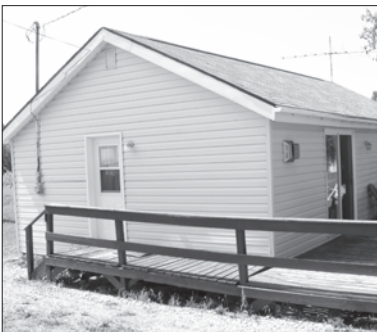
LAKE MANITOU COTTAGE on level lot w/60 ft. Rockville Road waterfrontage, sandy beach, good dock & sand bottom swimming. Bungalow 754 sq. ft. w/deck across water side has 2 bedrooms, 4 pc. bath, open kitchen dining living area w/propane stove fireplace. Recent upgrades of windows, doors, siding, shingles, fascia, soffits. Most contents including newer washer, refrigerator, stove. $154,000 (1431)
