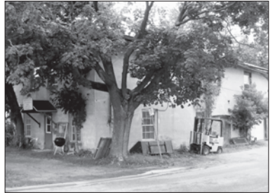
BLACKSMITH CENTRE on corner of Main & Meredith Streets w/4320 sq. ft. over 2 floors. Concrete building 36x60 ft. on fully serviced 39x127.6 ft. lot zoned core commercial. First floor garage plus business space & second level 4 & 1 bedroom apartments. $119,000 plus HST (1432)
