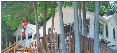
WATERFRONT HOME OR COTTAGE OFFERING great easterly views of the East Bluff on Gore Bay. Short distance to downtown. Master bedroom has a walk-in closet. Primary heat source is in-floor electric heating (3 zones), but there is also a gravity fed oil stove. $215,000. MLS#1033014
