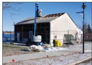
Demolition begins on the OPP boathouse in Little Current.
