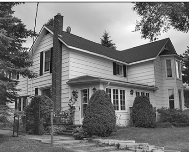
CENTURY HOME - In Little Current within walking distance to downtown and all other amenities. Adjoining lot included in the purchase price. This house has 4 large bedrooms and 2 bathrooms. Large double parlour on the main floor is ideal for entertaining and perfect for the home theater system. Spacious kitchen with adjoining dining room, main floor laundry. New windows, shingles, basement insulation with waterproof "drytrek", sump and dehumidifier all in 2011. $242,000. MLS#1027239
