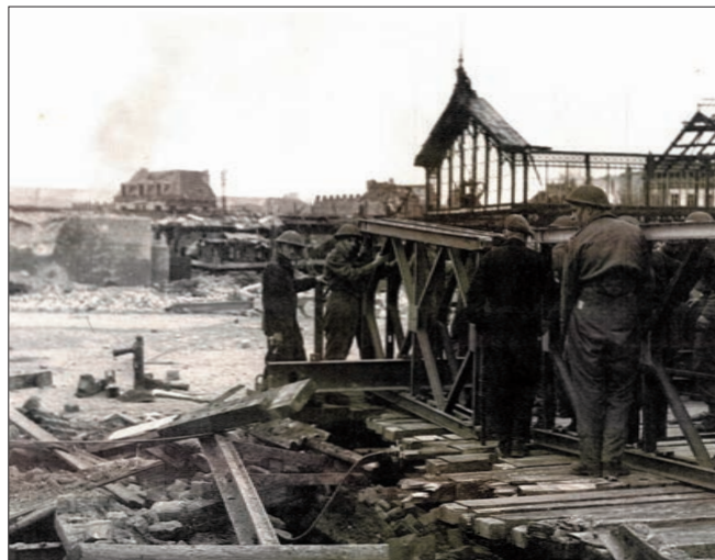
Royal Canadian engineers building a bridge day and night in Boulogne-sur-mer. September 18, 1944.
