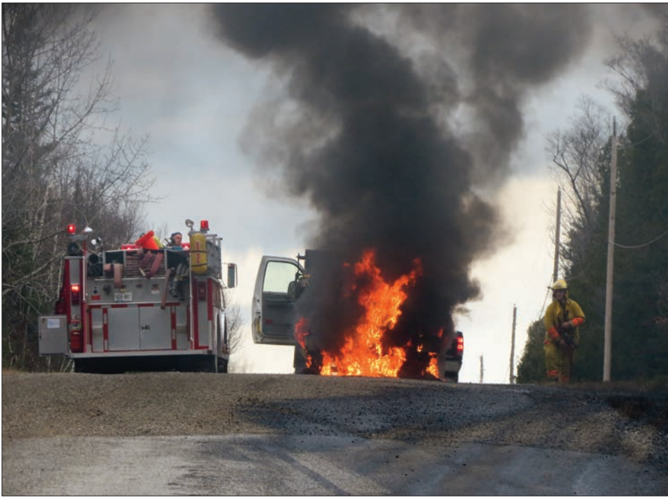
A tar kettle burns furiously on Government Road in Tehkummah as the fire department arrives to quell the flames.
