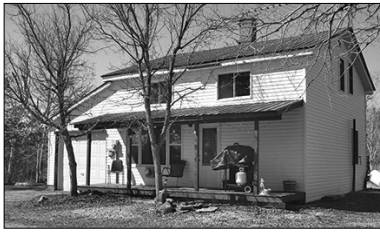
COTTAGE ON ACREAGE - A comfortable cottage on 90 acres fronting on a year round road. 24ft. x 24ft. on the main level plus an attached 12ft. garage/shop. It has been used as 4-season home. It recently was serviced with Hydro (underground), but can operate off-the-grid with the solar system and generator. Gravity fed water source for sink and toilet. 12V pump for shower. There is also a hunt cabin, small sugar bush, and seasonal stream. $149,000. MLS1024304
