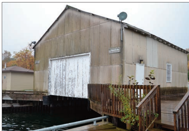
The old Little Current OPP boathouse is to be demolished next month.
