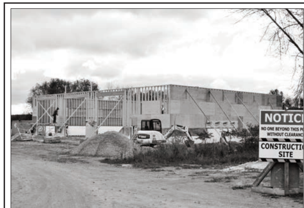
Construction underway on new public works building
