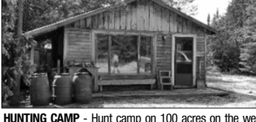
HUNTING CAMP - Hunt camp on 100 acres on the west end of Manitoulin Island. New propane stove. 1200 Watt generator and sauna included. Prime hunting area! $89,000. MLS#1020916
