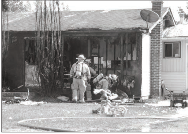
The Haggart family home was destroyed by fire last Friday afternoon. Thankfully, the family of four was not home at the time of the blaze.
