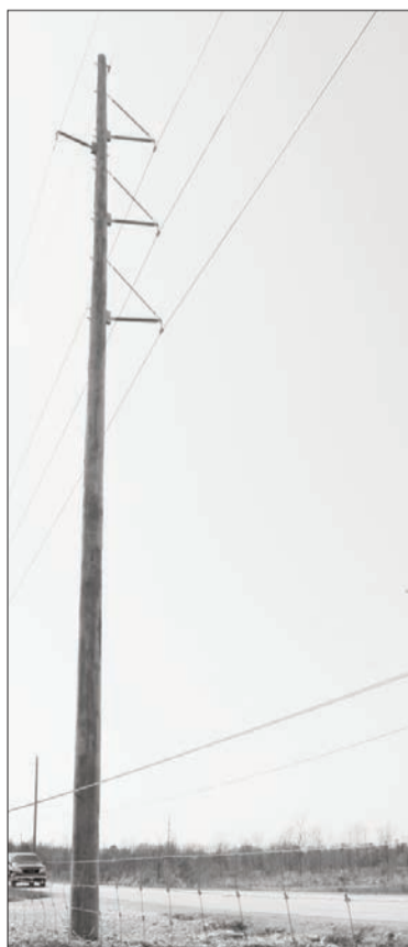
Craig Timmermans' electronic fence along Harbour View Road was energized through induced energy by the PowerTel lines running parallel, above his fence.
