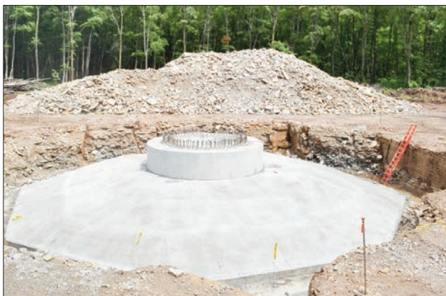
BELOW: The rebar frame is covered in cement and then backfilled.
