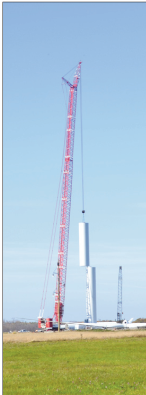
Section three of the tower in mid air.
