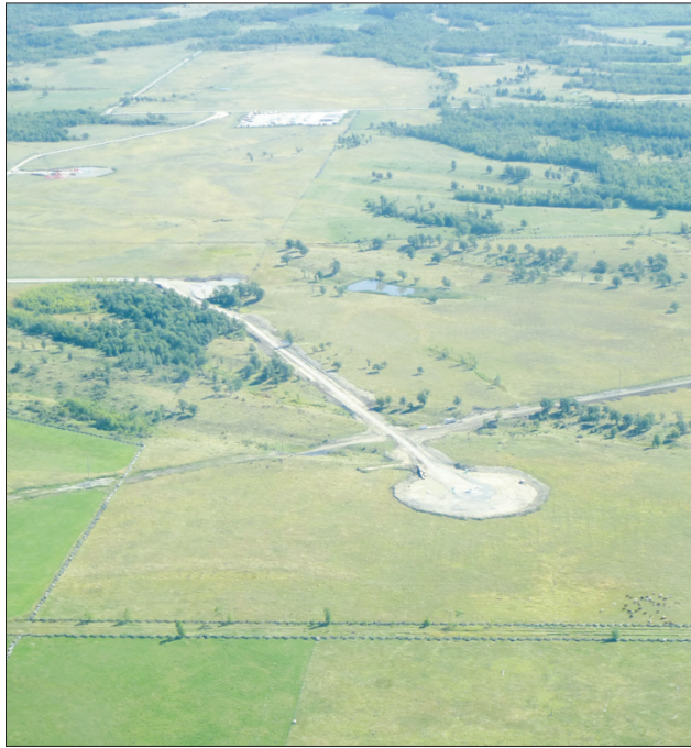
A view from the sky. This photo shows the area cleared for the T5 site.
