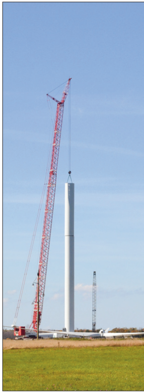
Section four of the T5 tower is carefully lowered into place.
