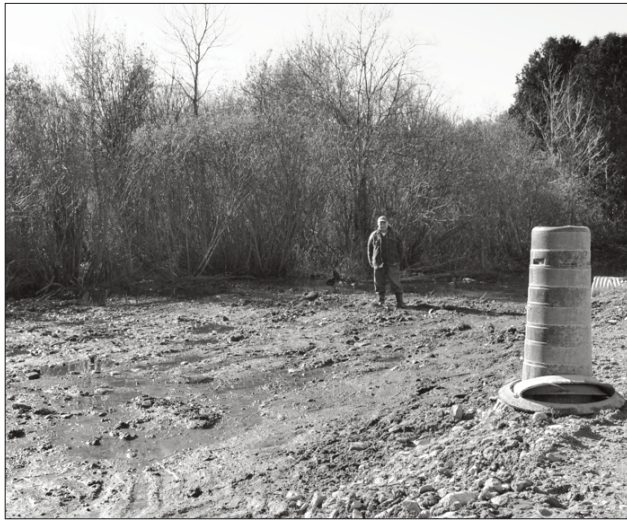
Green Bush resident Fred Delabbio stands next to the road where a 365-ton crane overturned on his property, spilling oil and breaking his fence.
