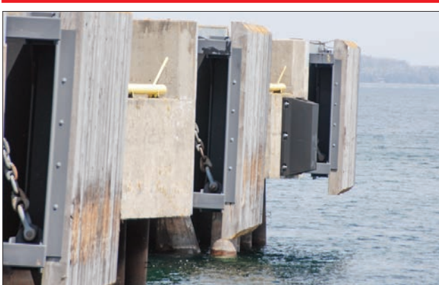
This docking pier at South Baymouth awaits Transport Canada improvements to mitigate low water so the Chi-Cheemaun can dock.
