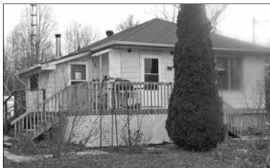
COUNTRY HOME just north of Sandfield on 0.56 ac. w/125.8 ft. highway frontage. Bungalow 854 sq. ft. on full basement w/2 bedrooms, 4 pc. bath, kitchen, dining & living rooms plus side entry mud room, south facing deck, 4 appliances & new oil furnace 2007. $79,000 (1050)
