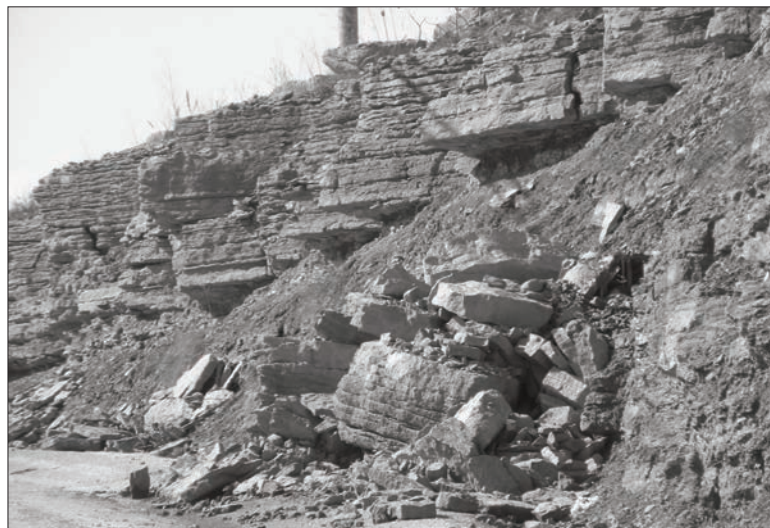
A pile of fallen rock gives lie to the original assertion that erosion would cause such rockfalls. Then town roads superintendant Garry Miller was vindicated.
