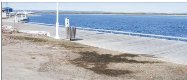
A leak of hydraulic oil had some Little Current residents concerned recently, but Northeast Town staff assure the spill was cleaned before seeping into the soil, or the water.
